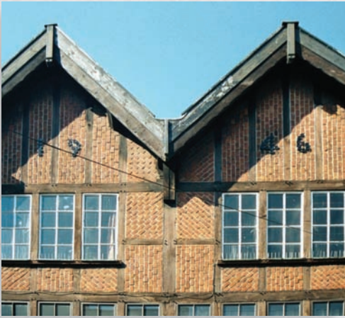
Above: Timber-frame building constructed in 1946 to replace a building destroyed by bombing in World War II. The 1946 date shown in the gables is made of bottle ends, Norwich, Norfolk, England.
