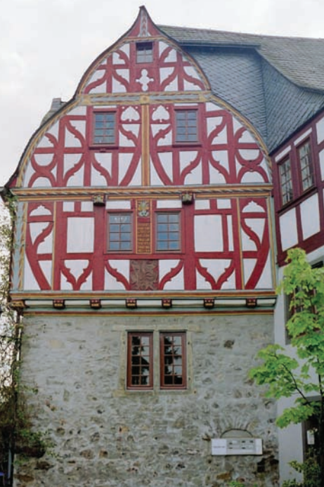
Left: House with stone lower story and timber-frame upper part with “man” pattern and cross, Limburg, Germany
